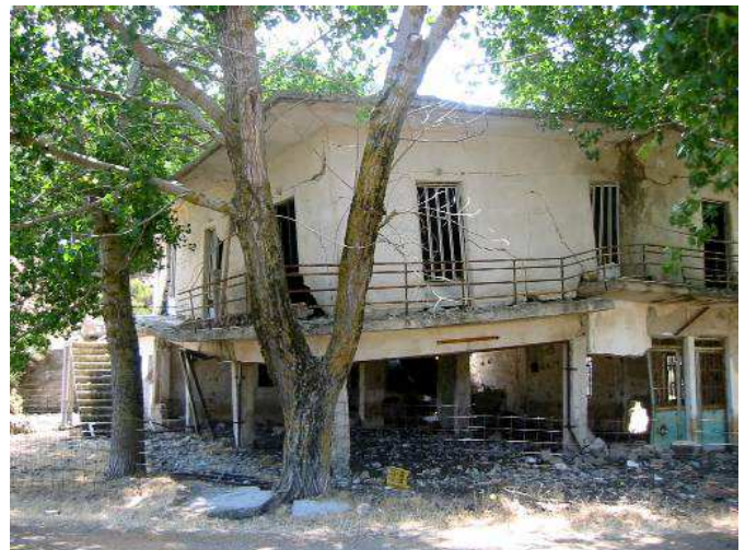
Pictures are showing views of a house on the western edge of the Omalos Plateau damaged during the quake of 1994
