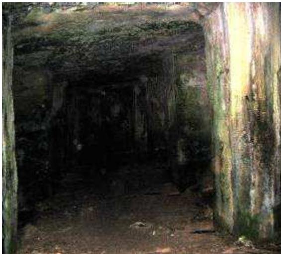
View into the cistern chambers: the single areas gain scales of approx. 40 x 20 m. In the vicinity of the entrance, the green colour of the pillars mark an algae growth through continuous moisture and twilight, under which the soft limestone suffers and loses "stability". Fotos: H. Eikamp (9/2004)
