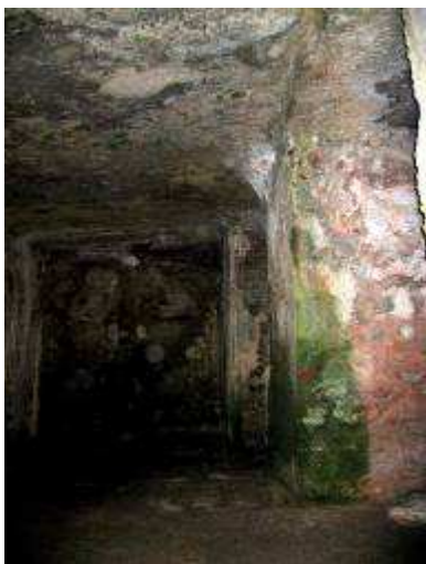
View into the cistern chambers: the single areas gain scales of approx. 40 x 20 m. In the vicinity of the entrance, the green colour of the pillars mark an algae growth through continuous moisture and twilight, under which the soft limestone suffers and loses "stability". Fotos: H. Eikamp (9/2004)
