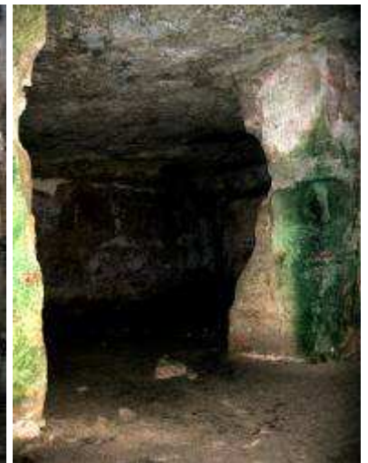
View into the cistern chambers: the single areas gain scales of approx. 40 x 20 m. In the vicinity of the entrance, the green colour of the pillars mark an algae growth through continuous moisture and twilight, under which the soft limestone suffers and loses "stability". Fotos: H. Eikamp (9/2004)
